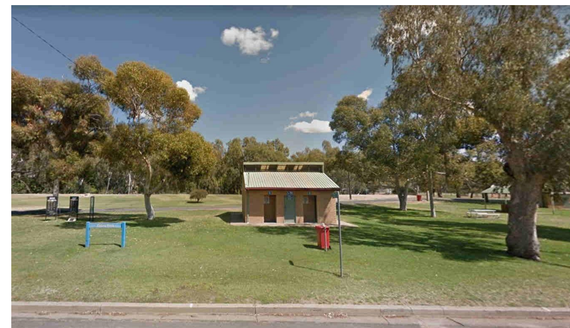
View from Oxley Hwy - Rest Area (toilets)
