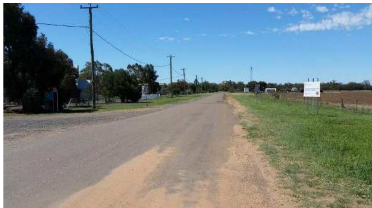
Coonamble St (street tree plantings & drainage upgrades)
