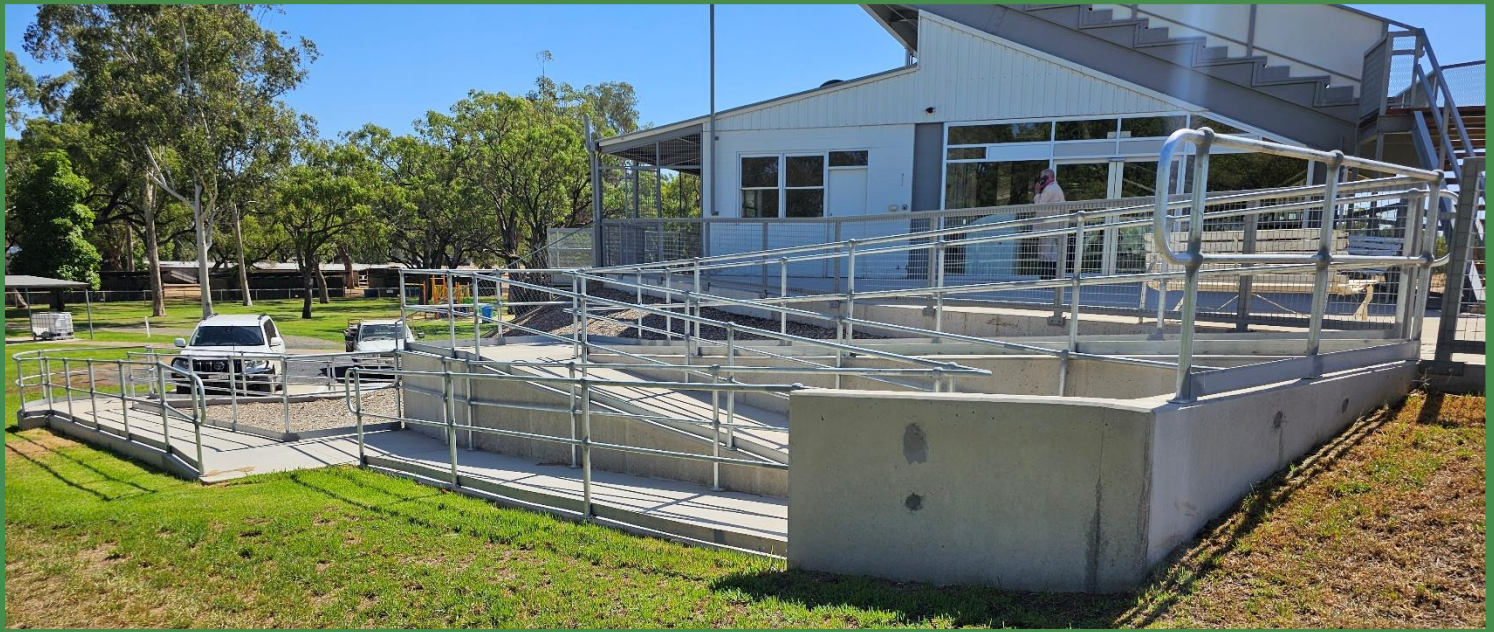
Showground/Racecourse Disability Access Ramp to GBS Falkiner Lounge
