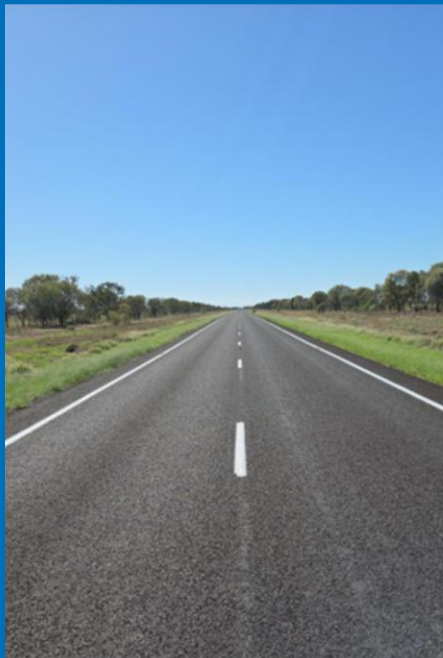
Heavy Patch Work on SH 11 Oxley Highway
