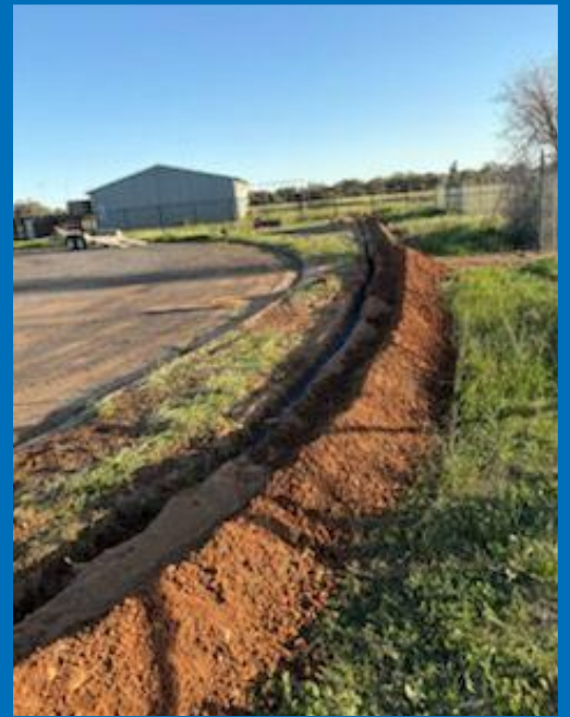
Water Mains Repairs and Maintenance
