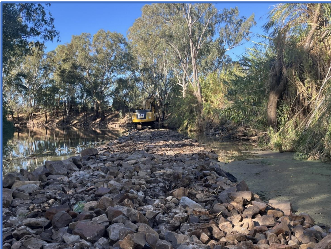
Warren Town Levee Rehabilitation Works
