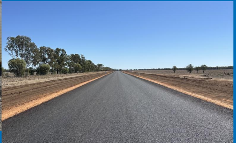
Working on the RR202 Marthaguy Road as part of the Towards Zero Safety Roads Program.
