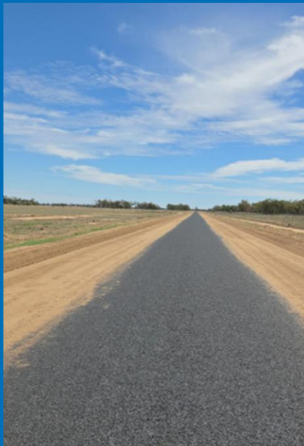
Shoulder Grade on SR 65 Old Warren Road
