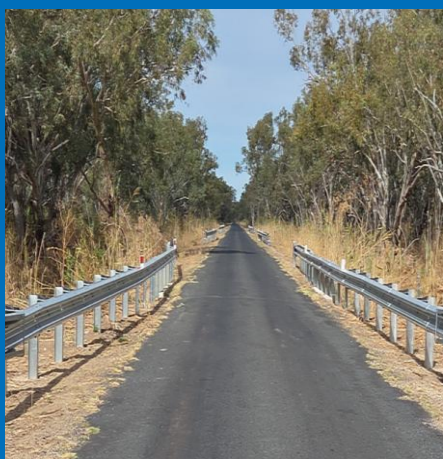
Guardrail Replacement on Ginghet Swamp Bridges on RR333 Carinda Road
