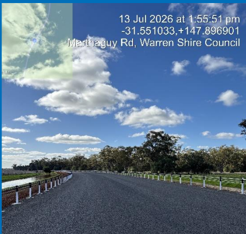
RR202 Marthaguy Road Safety Wire Ropes
