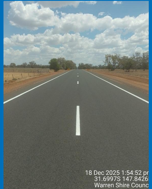
Warren Road Rehabilitation
