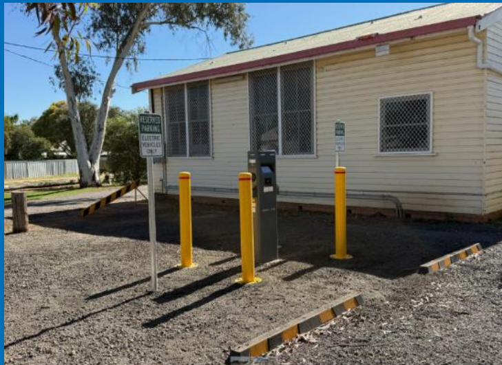
Warren and Macquarie Marshes Visitor Information Centre EV Charging Station
