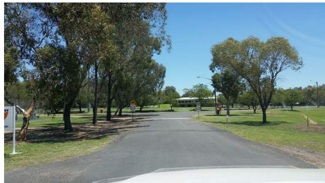
Main driveway looking west towards Victoria (main) Oval
